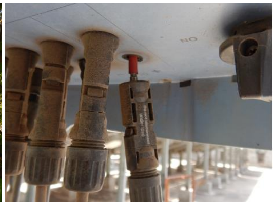
Figure 63: Loose connectors in the inverter inputs
