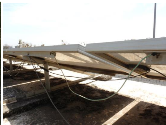
Figure 149: Equipotential bonding (cable management)
