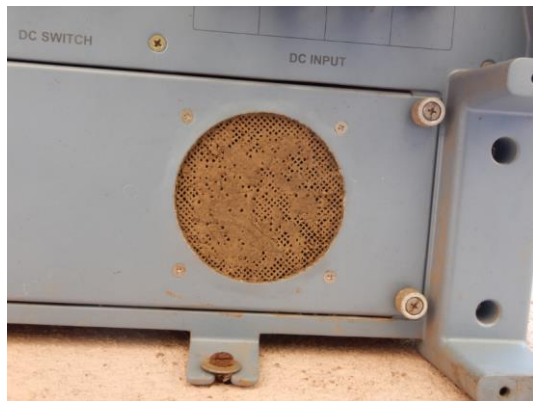
Figure 94: Inverter fan filters (outlet) partially blocked
