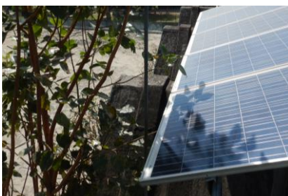
Figure 27: Near shading by trees
