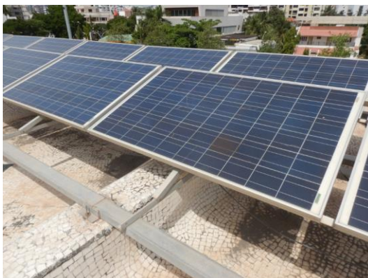
Figure 150: Advanced cell degradation (temperature)
