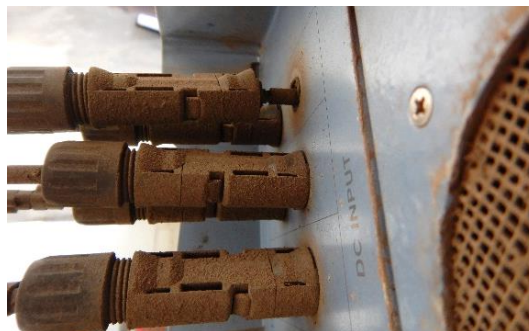
Figure 78: Broken connectors on inverter
