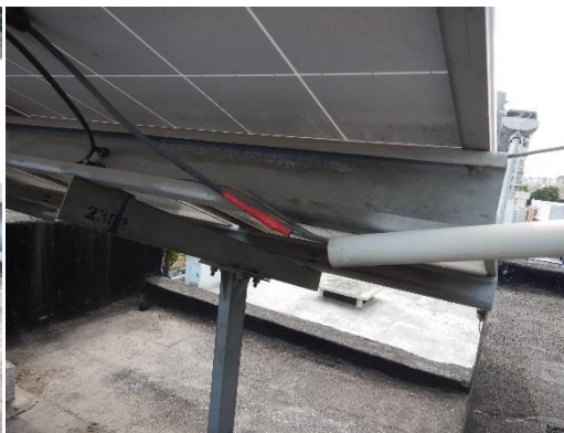
Figure 51: Cables connected with duct tape
