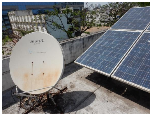
Figure 111: Shading from antenna
