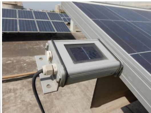
Figure 140: Irradiation sensor – plane of array
