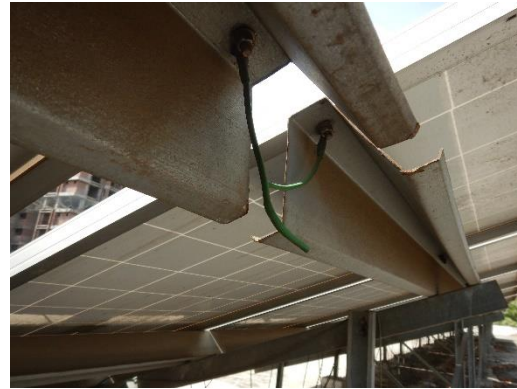
Figure 120: Broken ground wire
