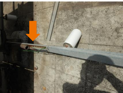
Figure 113: Broken cable ducts
