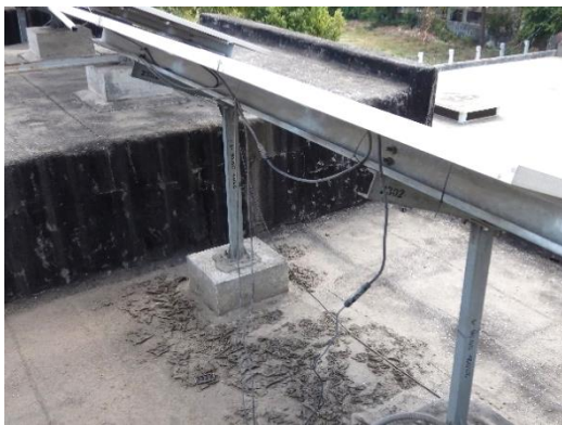
Figure 50: Loose hanging cables
