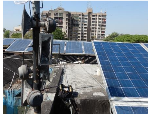
Figure 32: Shading by objects in the building
