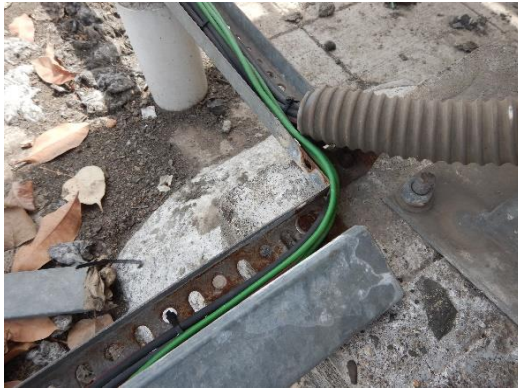
Figure 119: Non-functional grounding
