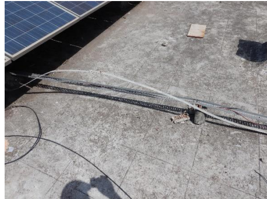
Figure 105: Open and broken cable ducts
