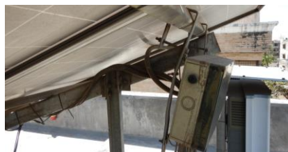
Figure 70: Improper attachment - combiner box
