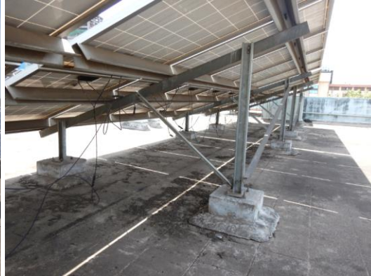
Figure 134: Fixed tilt mounting structure foundations
