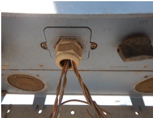
Figure 123: Poorly installed sensor cables
