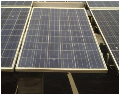
Figure 84: String with module with broken glass
