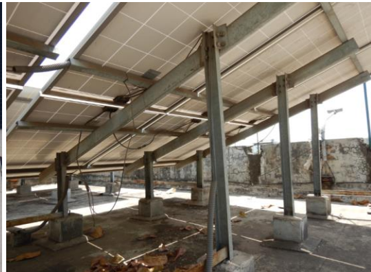
Figure 65: Cables in contact with sharp edges
