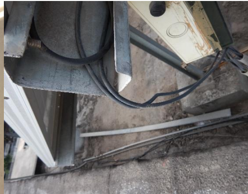
Figure 47: Cables in contact with sharp edges
