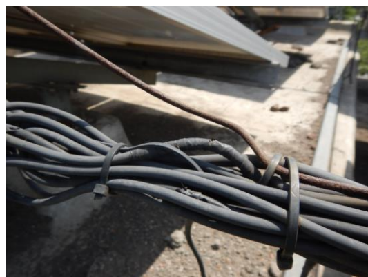
Figure 19: Cable management (damaged/bending)
