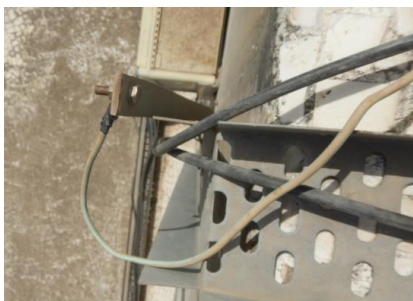
Figure 142: Damaged cables: sharp edges
