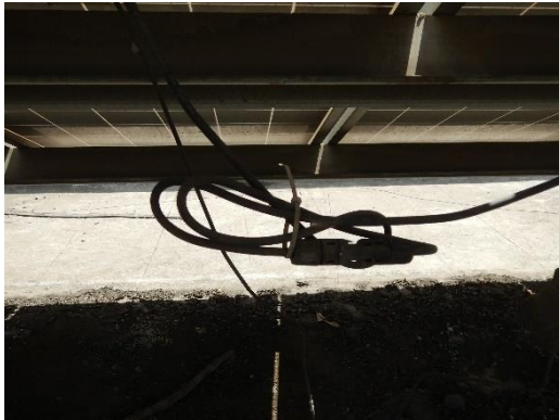
Figure 104: Critical bending radius
