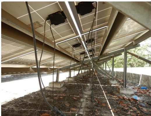
Figure 121: Loose/hanging cables
