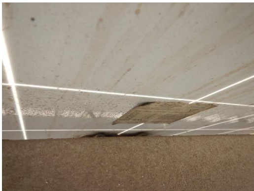
Figure 106: Module label issues
