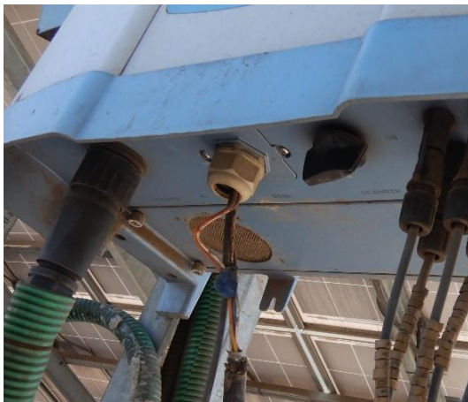
Figure 80: Broken sensor wiring
