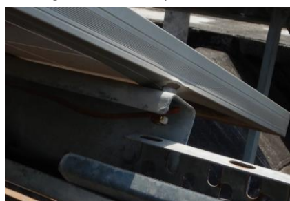
Figure 24: Screws of the fastening clamps
