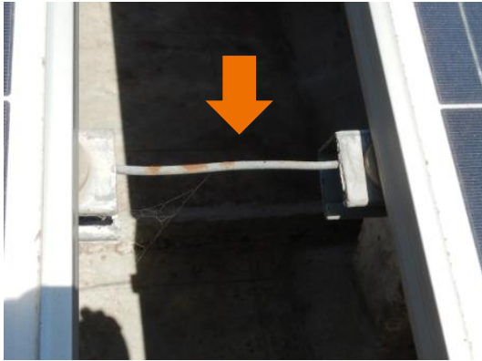
Figure 76: DC cables exposed to UV radiation
