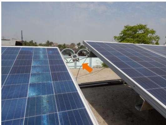
Figure 22: Improper installation of reference Si-sensor
