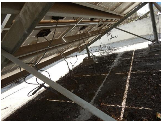
Figure 108: Loose hanging cables
