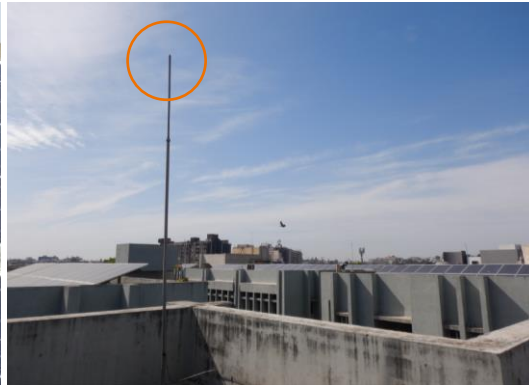
Figure 138: Lightning arrester without spikes
