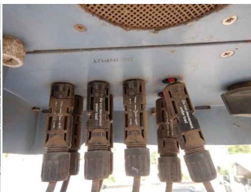
Figure 53: Broken MC connector
