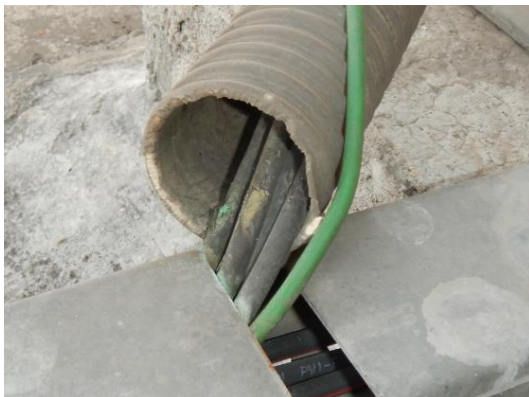
Figure 139: Cables damaged by sharp edges
