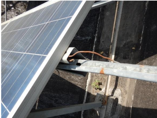
Figure 31: Non-functional grounding
