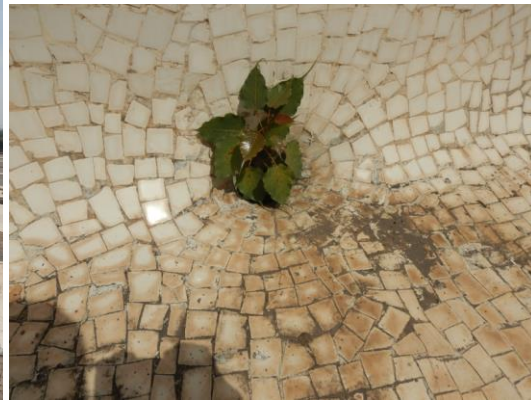
Figure 147: Drainage partially blocked
