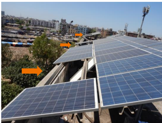
Figure 91: Strings in open circuit (broken modules)
