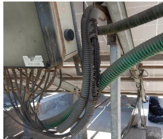
Figure 81: Broken cable duct
