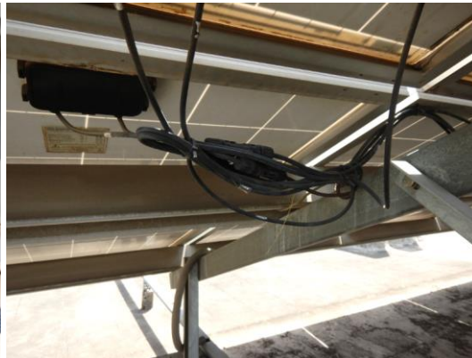
Figure 136: DC cabling management
