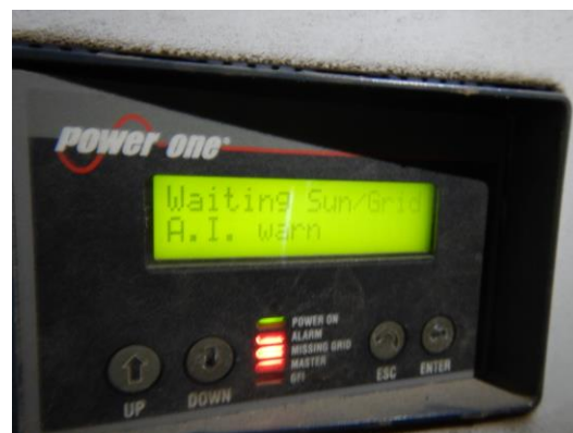
Figure 152: Inverter status (waiting sun/grid)
