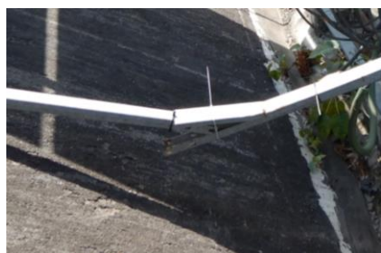
Figure 25: Broken cable ducts
