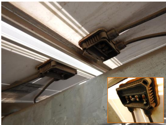
Figure 66: Modules with open J-boxes (ca. 40%)
