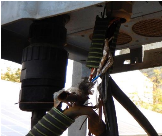
Figure 35: Broken sensor wiring
