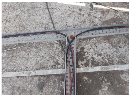
Figure 97: Cables in contact with sharp edge
