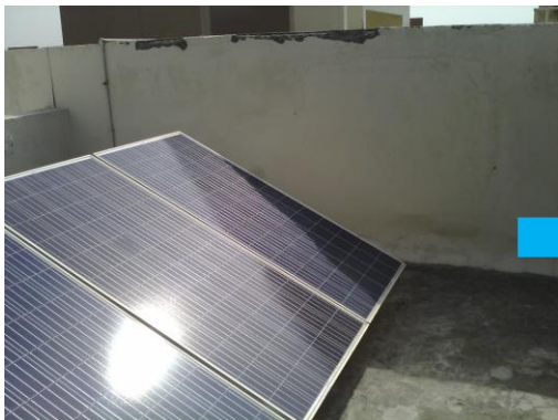
Figure 79: Near shading on the module surface (VI)
