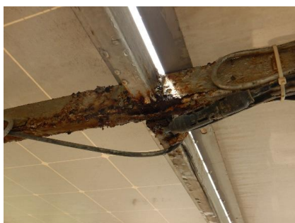
Figure 49: Rusted mounting structure
