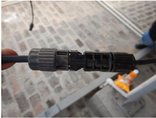
Figure 110: Open connectors
