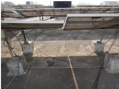
Figure 33: Inconsistent tilt
