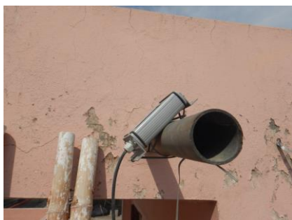
Figure 106: Inaccurate fixing of the sensors
