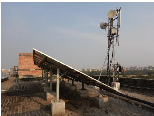
Figure 17: Near shadings on the PV surface
