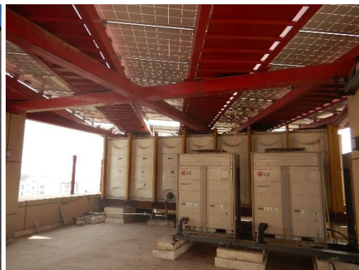
Figure 48: Mounting structure and module anchorage
