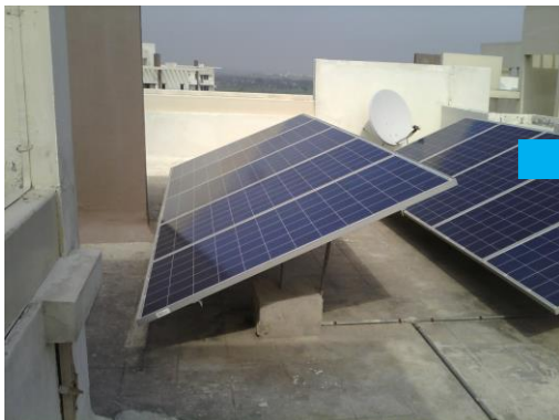
Figure 81: Near shading on the module surface (VI)
