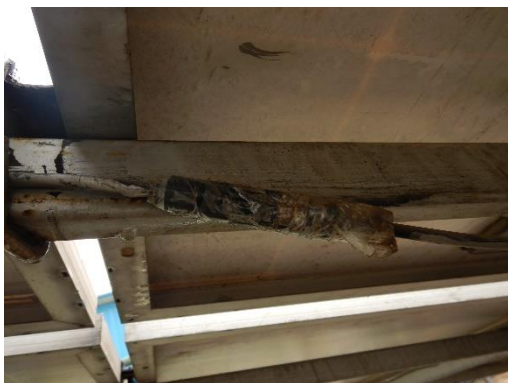
Figure 56: Inaccurate DC cabling
