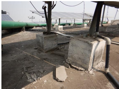
Figure 23: Weak foundations
