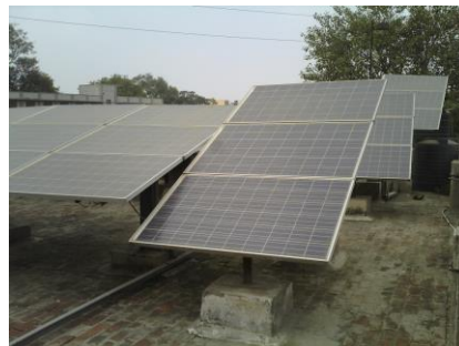
Figure 119: Inconsistent module tilt
