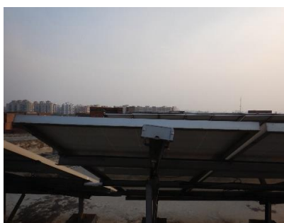
Figure 11: Irradiation sensor misaligned
