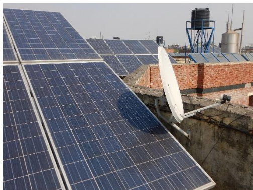
Figure 20: Near shadings on the PV surface
