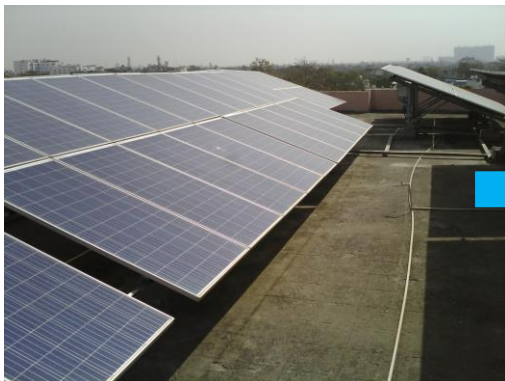
Figure 12: Near shading on the module surface (VI)
