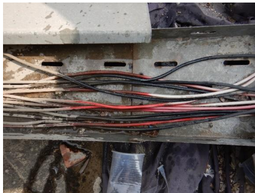
Figure 34: Inaccurate DC cable routing
