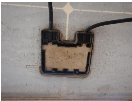
Figure 57: Junction box without lid
