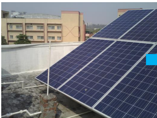
Figure 93: Near shading on the module surface (VI)
