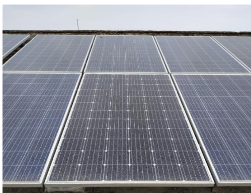
Figure 105: Mixing of poly and mono c-Si modules
