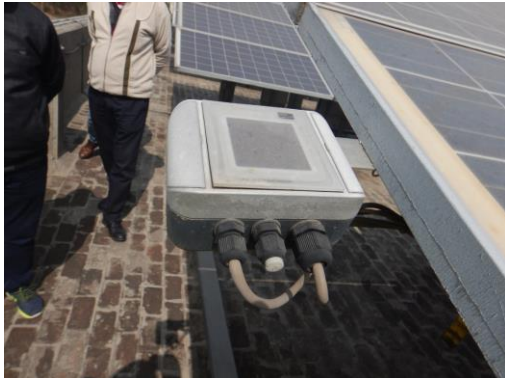
Figure 121: Dirty irradiation sensor
