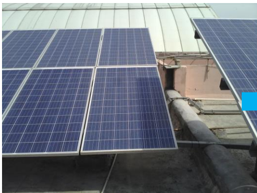
Figure 114: Near shading on the module surface (VI)
