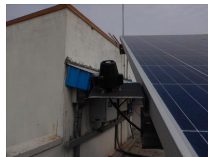
Figure 86: Irradiation sensor wrongly installed
