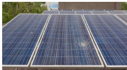
Figure 30: Broken module
