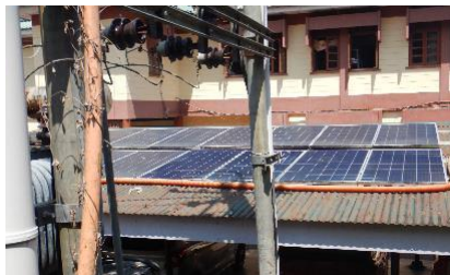
Figure 103: Shading from cables and poles
