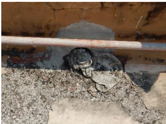
Figure 98: Blocked drainage
