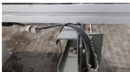
Figure 41: Broken tube (UV exposed)
