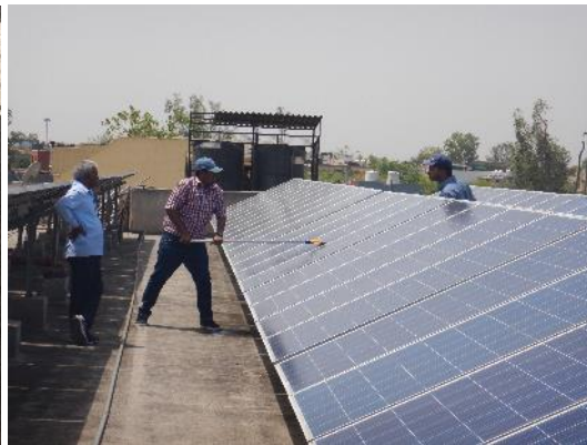
Figure 24: Cleaning of the modules
