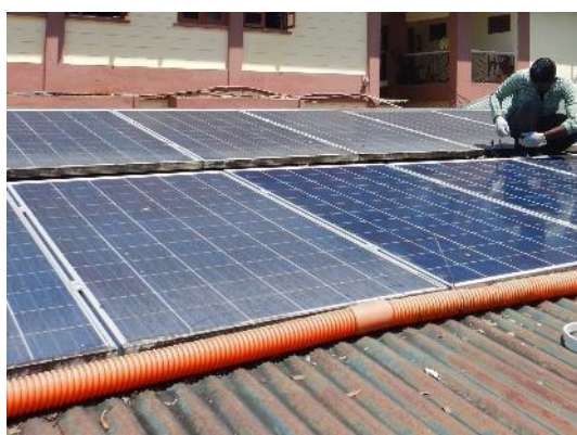
Figure 106: Dirty and clean modules
