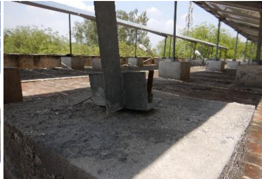
Figure 62: Loose fixation of the mounting structure
