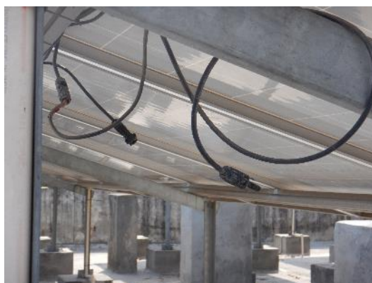
Figure 72: Connectors found disconnected
