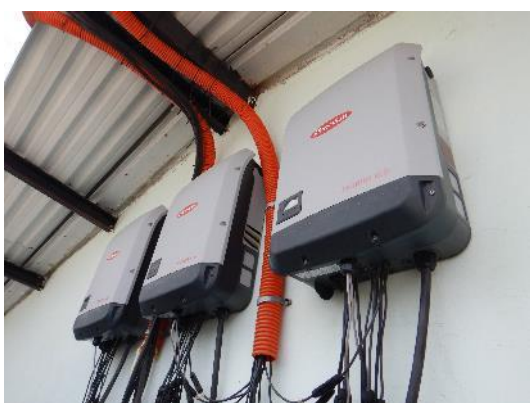
Figure 130: Inverters of the system
