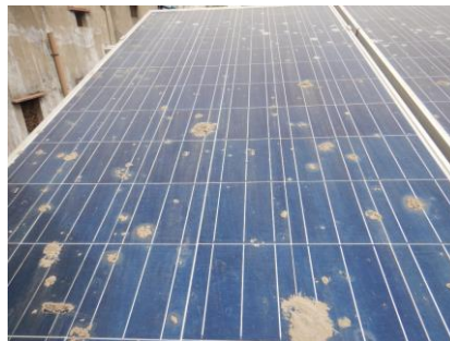
Figure 29: Soiling on the modules
