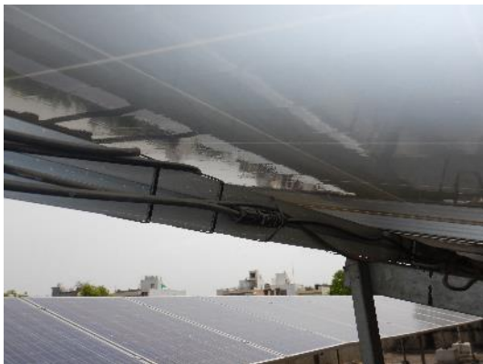
Figure 50: Cable fixation
