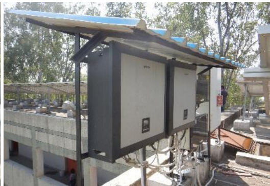
Figure 60: Inverters of the system
