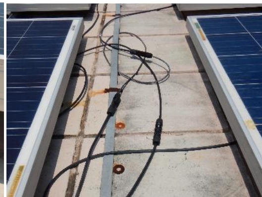
Figure 96: Connectors and cables exposed to UV
