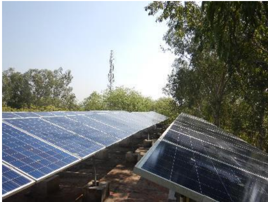
Figure 57: Trees cause significant shading
