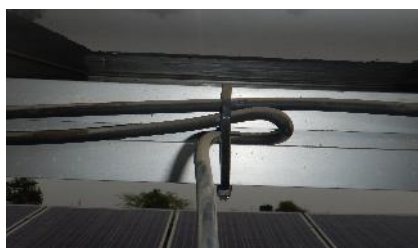
Figure 40: Small bending radius
