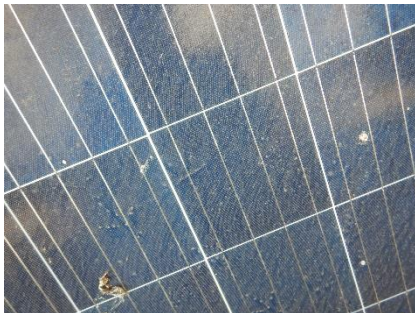
Figure 124: Heavy soil on the modules
