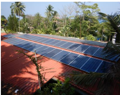
Figure 77: Near shading situation
