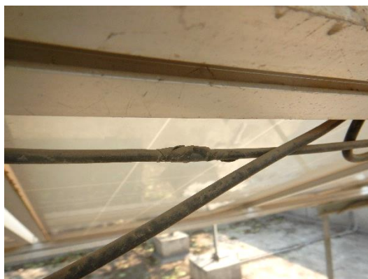
Figure 76: Damaged cable from sharp edges
