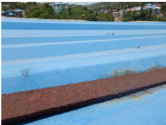
Figure 134: Rusty roof elements
