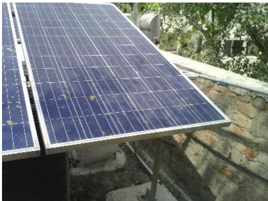
Figure 52: Warm cells caused by shading from trees, VI (left), IR (right)
