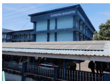
Figure 112: Modules are heavily soiled
