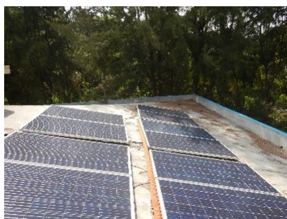
Figure 91: Shading from trees
