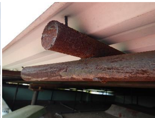
Figure 129: Rusty roof elements
