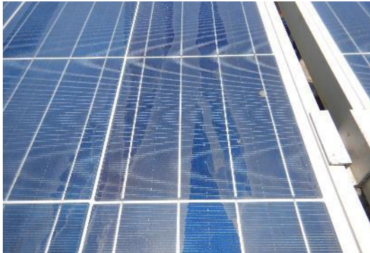
Figure 61: Soiling on the module surface
