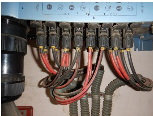
Figure 25: Connections at the inverter
