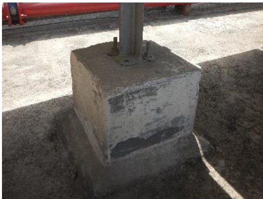
Figure 23: Foundation of the mounting structure
