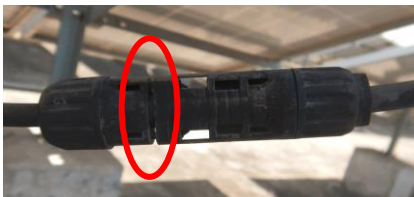
Figure 14: Connector not tightly closed
