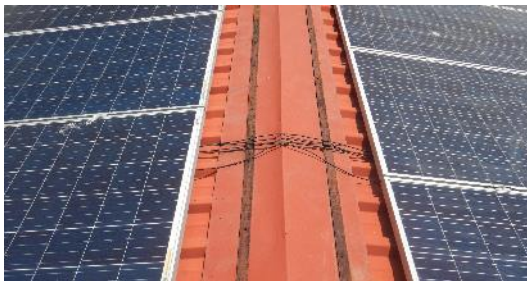
Figure 86: Cables exposed to UV radiation
