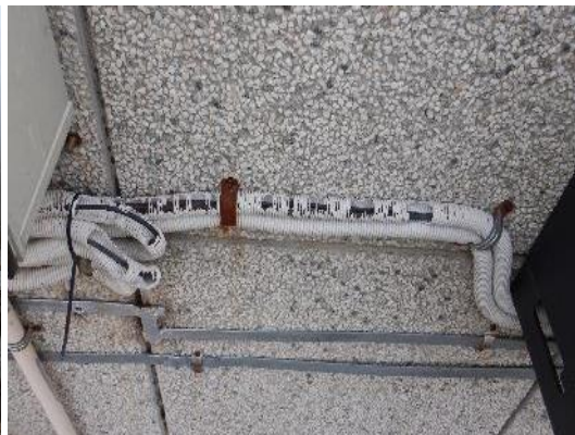
Figure 51: Broken tube
