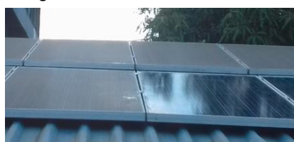
Figure 113: Severe soiling losses
