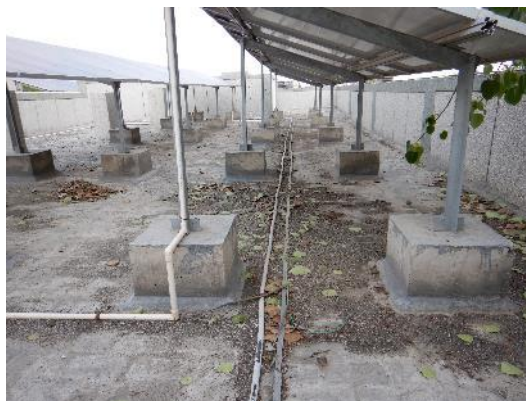
Figure 70: Foundation of the mounting structure
