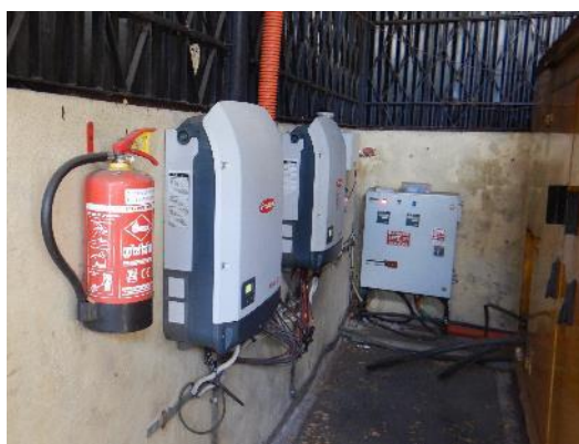
Figure 109: Inverters of the system
