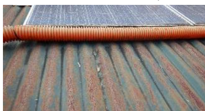
Figure 101: Rusty roof
