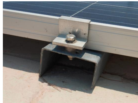
Figure 95: Loose fixation of a module
