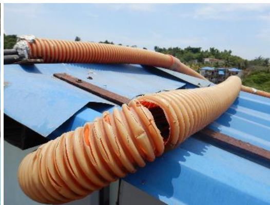
Figure 135: Broken protective conduit
