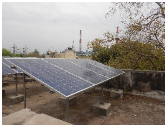
Figure 39: Trees causing shading
