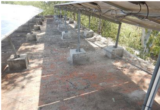
Figure 59: Foundation of the mounting structure
