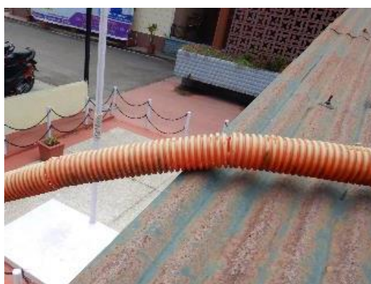
Figure 107: Broken protective tube
